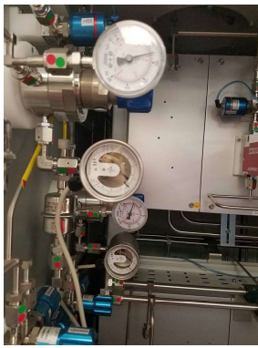
Figure 12: H 2 and N 2 sensors in the cabinet
