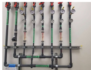
Figure 10: Cooling water pressure check
