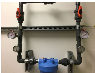
Figure 8: Water filter pressure difference check
